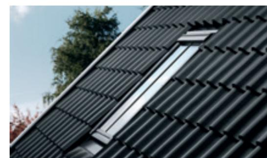
In addition to a glazing bar, you may be asked to install your roof window deeper into the roof than can be achieved with standard installation. To do this you should select a recessed flashing kit, streamlining the roof window so less protrudes above the roofline.
